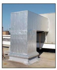
**Alumaguard® Lite** flexible weather-proofing cladding from **Polyguard Products** is one of the family of **Alumaguard** cladding products that offers superior cold weather performance, ease of handling and application and true zero perm performance
